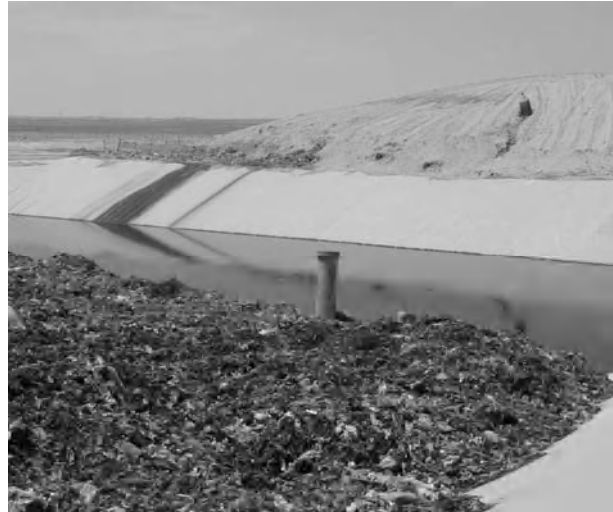
Fig. 1 Leachate generated from biodegradation of organic waste at a landfill site located in a desert. Note black and brown leachate stain due the leachate leaking from the adjacent completed cell (upper left) into the operating cell (foreground)
